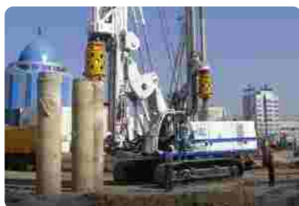
桩工 Pile Work
